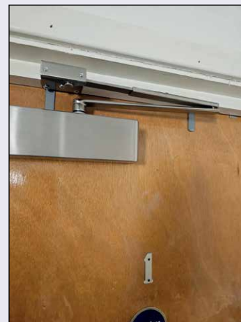
Students placing hooks for hanging clothes can lead to leaf, frame and seals damage.
