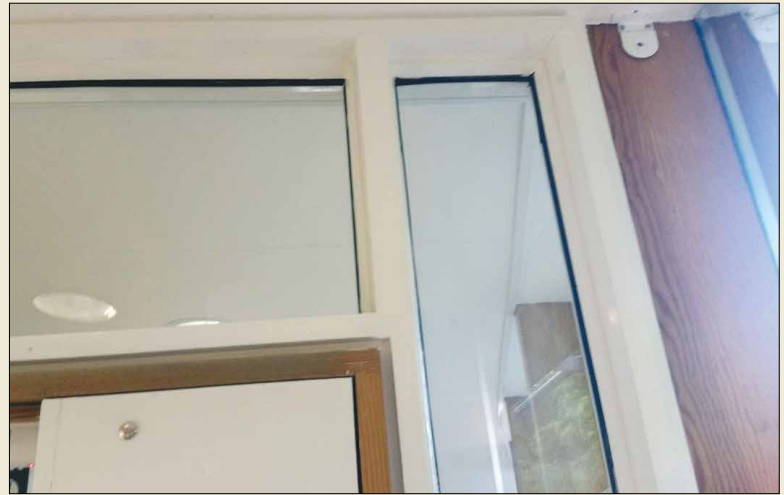
An example of a doorset with glazed overpanel and side panels.
