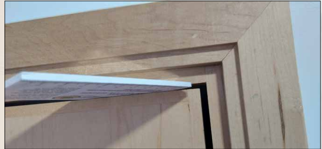
Checking if gaps are uniform and within tolerance.
