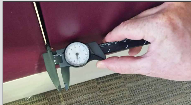
Checking a double door meeting gap with dial calipers during a Type 2 inspection.
