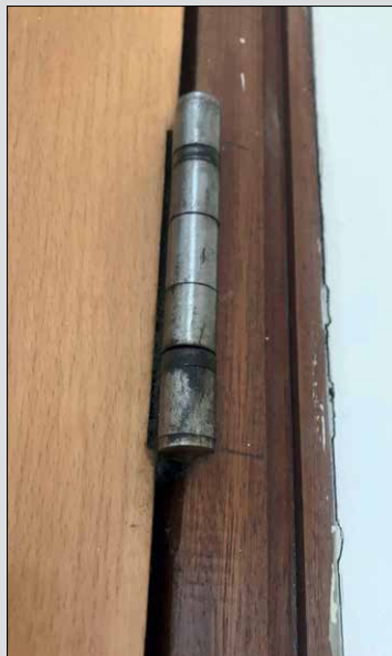
A hinge which has sediment buildup and grime due to lack of maintenance.
