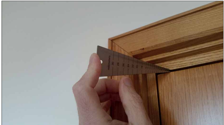
Checking the top edge of a door leaf during a Type 1 inspection.
