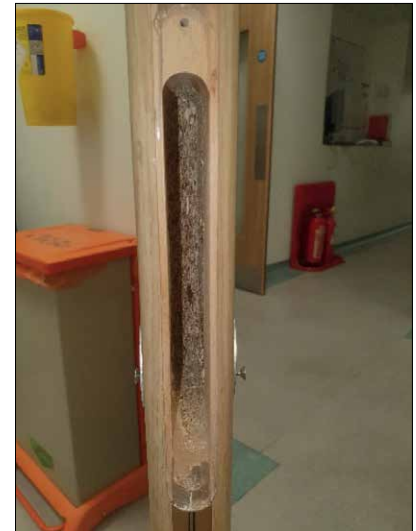
Removal of lock casing to identify the door leaf core construct.
